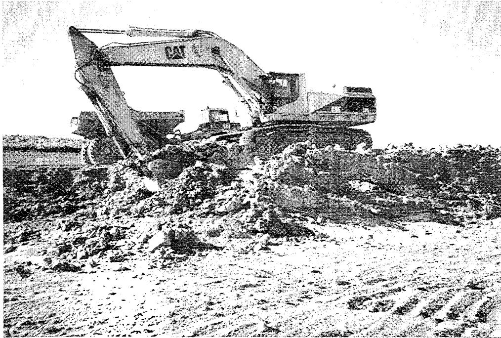
FIGURE 63 Soil Mixing during excavation
