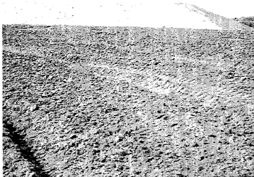
FIGURE 21 Embankment of A-2-4 material with moisture control
