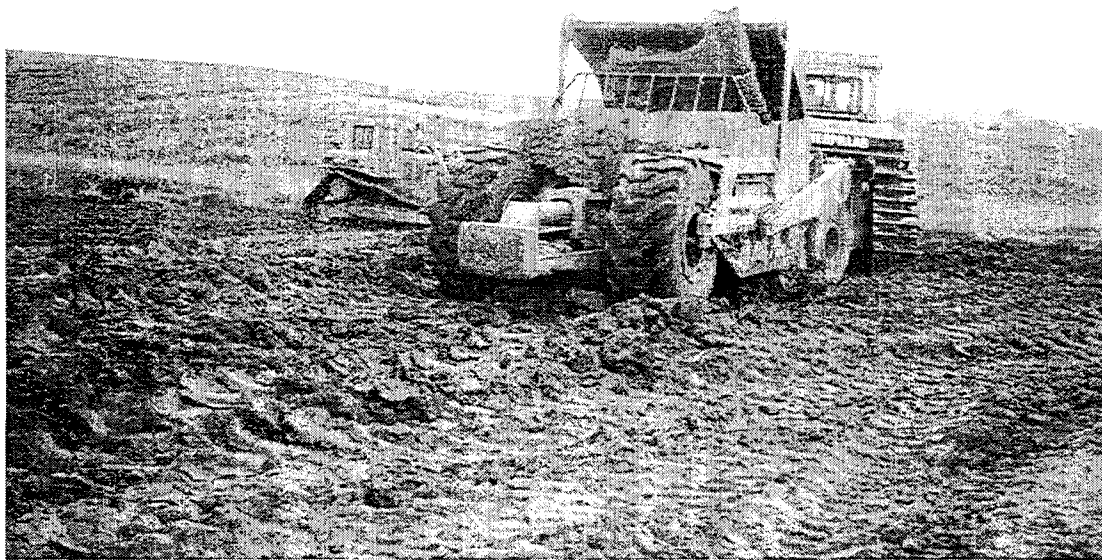
FIGURE 40 Organic material and large clods from scraper excavation
