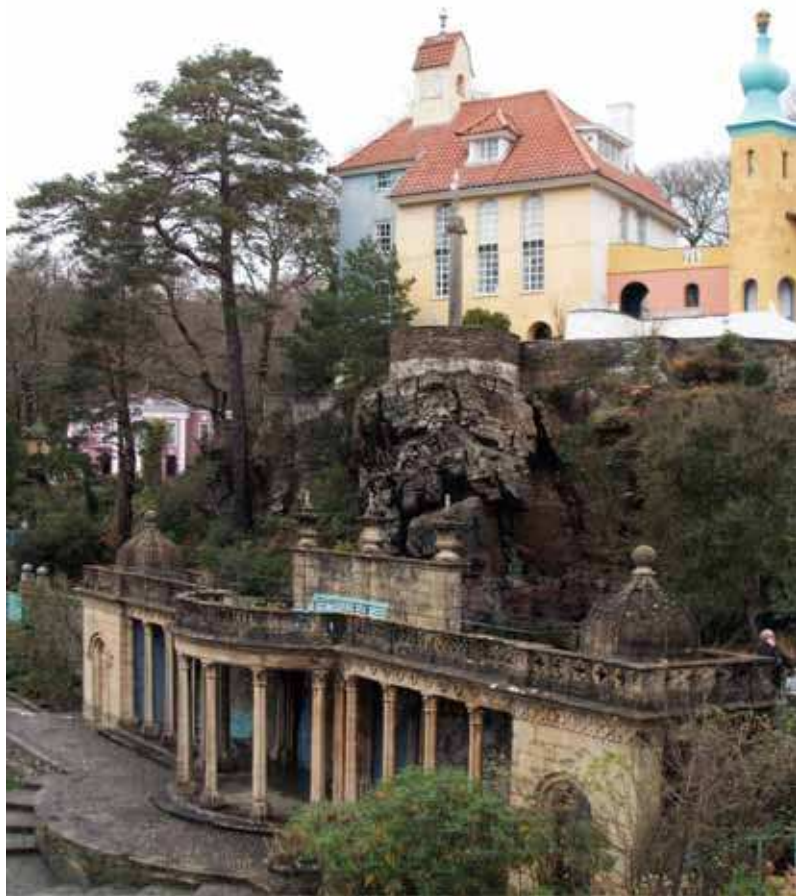
Figure 14: The Chantry, view from the Round House (photograph: F. Ellis)
