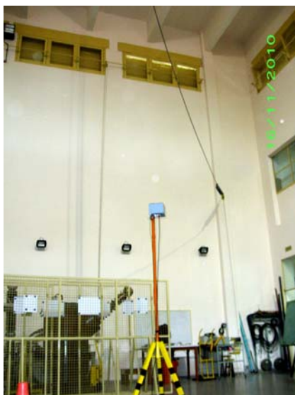
Fig. 2. EFS placed in the High Voltage Lab, under a cable fed with fundamental frequency voltage and Flicker.
