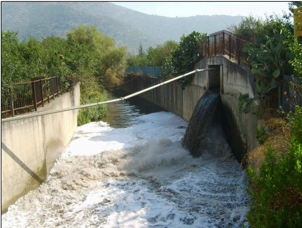
Fig. 3.8 - Outflow of Mercato San Severino treatment system (photo taken on August 2011)
