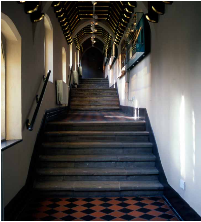
Fig 3. The cloister at A.W.N. Pugin's 1844 extension to his original Mercy Convent, Handsworth, in the West Midlands. Listed Grade II*. Photographed in 2006.
