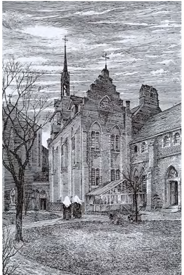
Fig 1. A.W.N. Pugin's Mercy Convent at Bermondsey, 1838 (demolished), his first purpose-designed religious community building, seen from the north-east and drawn for the Architectural Review in the 1890s by Francis D. Bedford.
