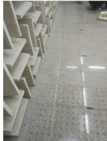
FIGURE 7: Scene of laying fiber.
