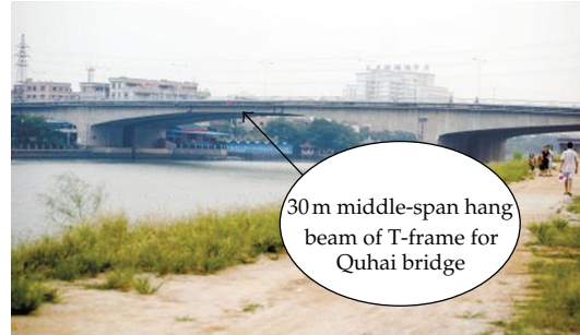
Figure 1: A photo of Quhai T-frame bridge.
