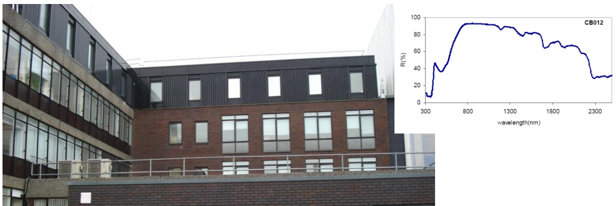
Figure 2: External view and spectral characteristics of the cool roof paint for the case-study building in London.
