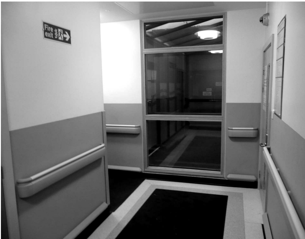
Fig 6. Corridor to right of door.
