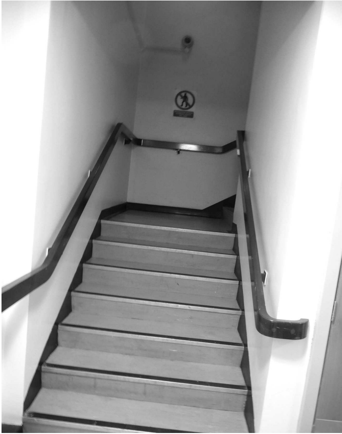
Fig 5. Stairs with 'No Entry' sign
