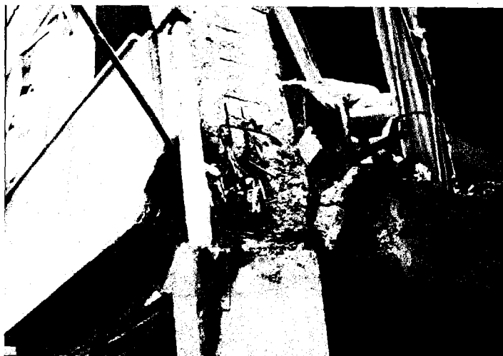
Figure 1.1: Damaged beam-column joint during earthquake (1999 Kocaeli, Turkey)
