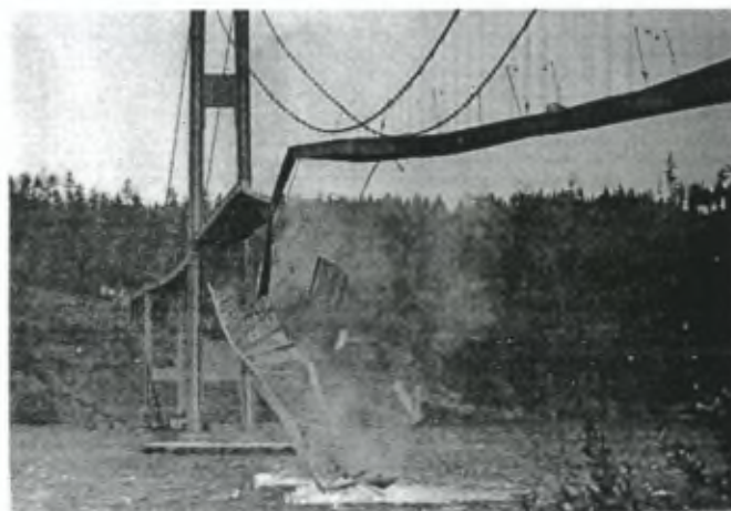
Figure 1.3: Failure of the Tacoma Narrows bridge by torsion flutter at a wind speed of 42 mph in 1940.
