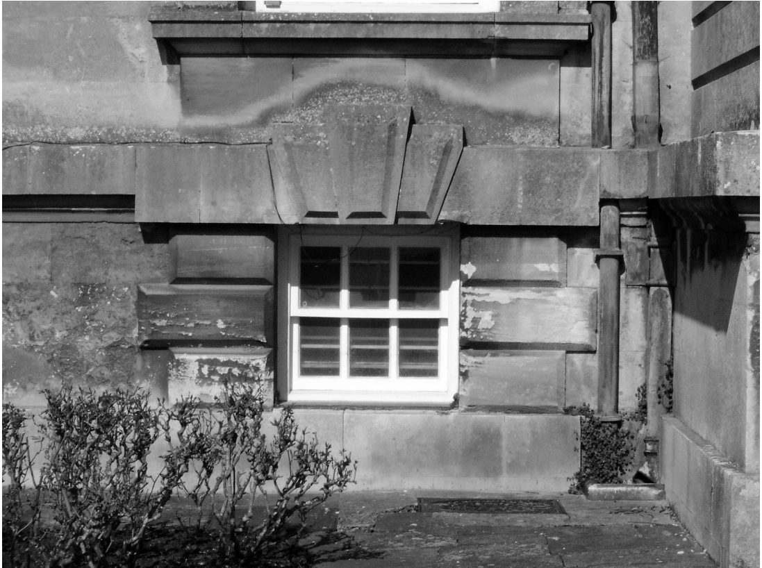
Fig. 68 Basement Window, South Front of Blenheim Palace , showing the revised design as used for twelve of the original twenty-four south front basement windows when the front was extensively rebuilt in early 1707
