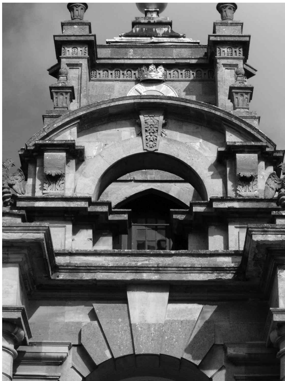
Fig. 85 View of Kitchen Wing Tower, Blenheim Palace, from the West
