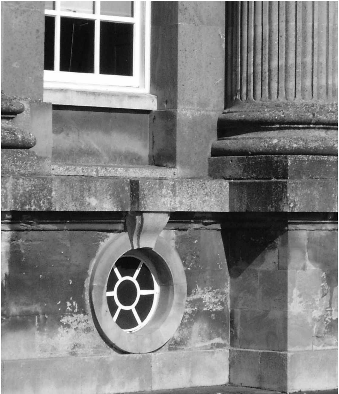
Fig. 67 Basement Window, South Front of Blenheim Palace , showing the original circular design initially used for all the basement windows
