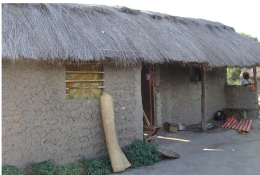
Figure 3 Local huts. Local houses in the study area are constructed with corrugated iron sheets or thatched roofing and the walls are constructed with bricks or mud. Most houses are rectangular in shape and have open eaves.
