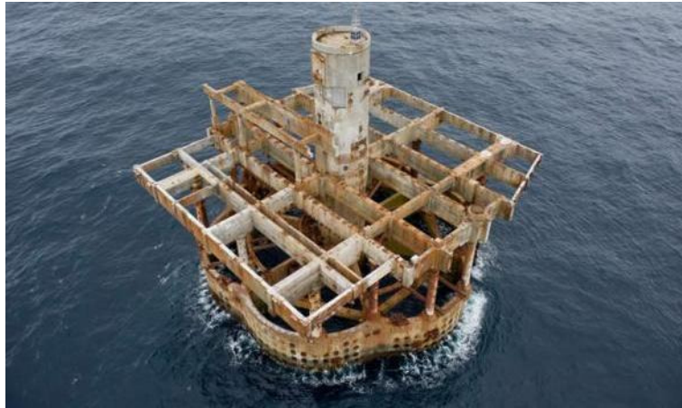
FIGURE 2.3 DECOMMISSIONED MCP01 PLATFORM (TEP UK, N.D.)
