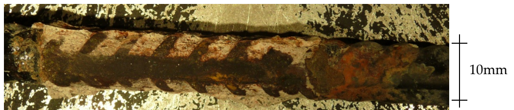
FIGURE 5.17 RED/BLACK CORROSION PRODUCT (OXYGENATED WATER)
