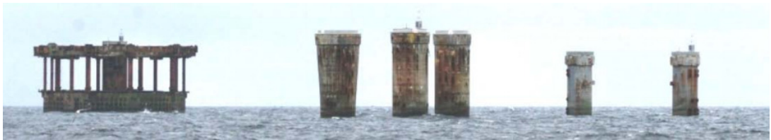
FIGURE 2.4 FRIGG CDP1, TCP2 AND TP1 AFTER DECOMMISSIONING (TOTAL E&P NORGE AS, 2011)
