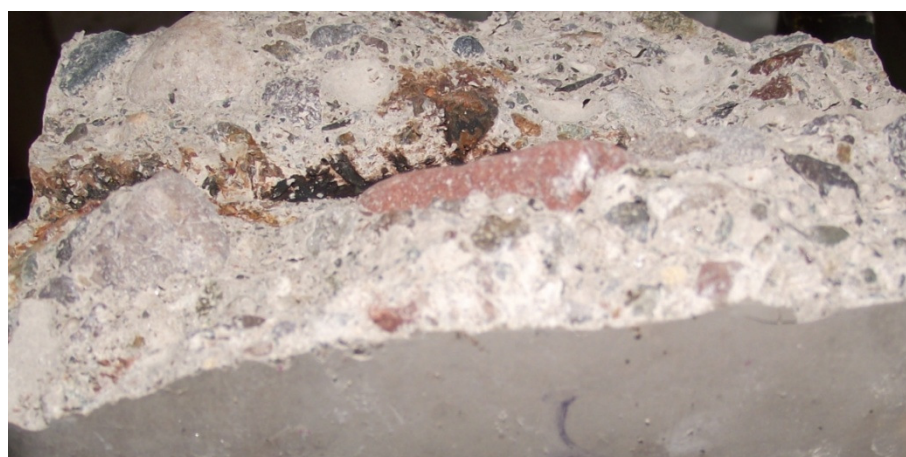
FIGURE 5.18 MINIMAL RUST STAINING (ATMOSPHERIC)
