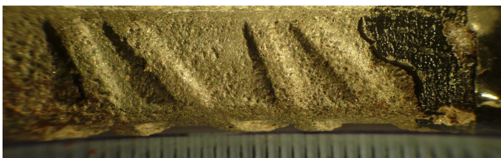
FIGURE 5.21 CORRODED REINFORCEMENT FROM BEAM C1
