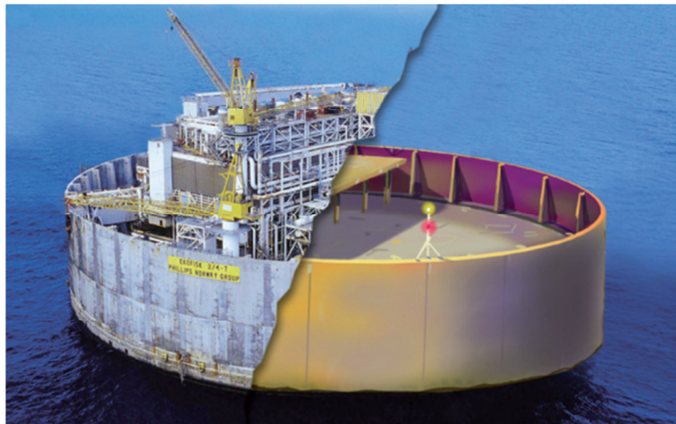
FIGURE 2.5 EKOFISK TANK BEFORE/AFTER TOPSIDE REMOVAL (NORWEGIAN PETROLEUM DIRECTORATE, N.D.)
