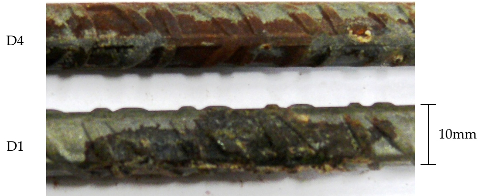
FIGURE 5.5 COMPARISON BETWEEN CORROSION PRODUCTS ON ANODES IN BARS D4 (TOP) AND D1
