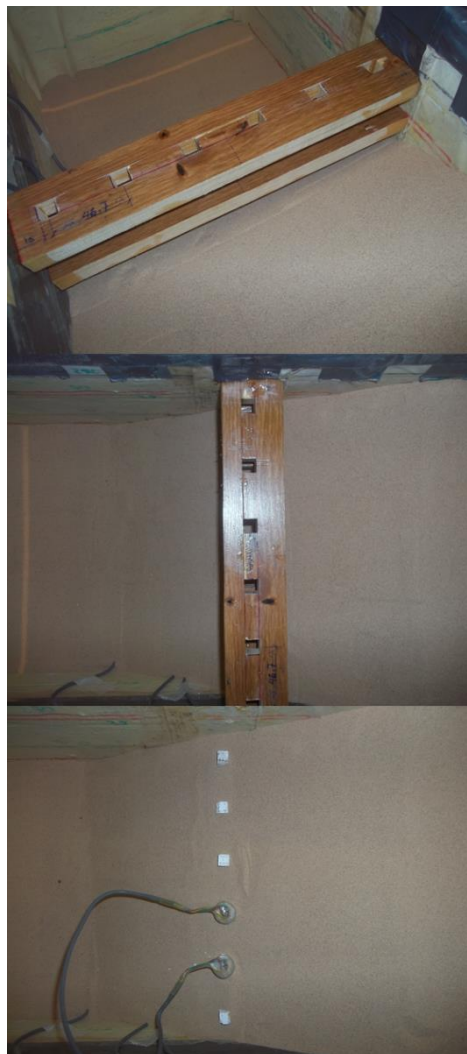
Figure (3- 38): Perforated wooden jigs and resulting installed piles ( s = 4.67B shown)
