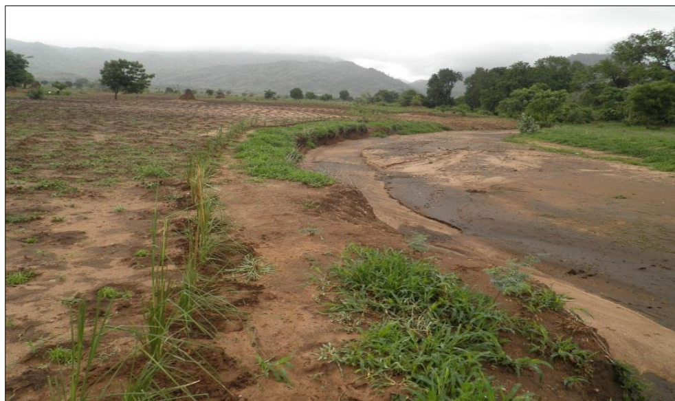
Figure 4-3: Vertiva grass being used to reduce impact of flooding on crops. Without protection, fields are reduced in size by river action every year
