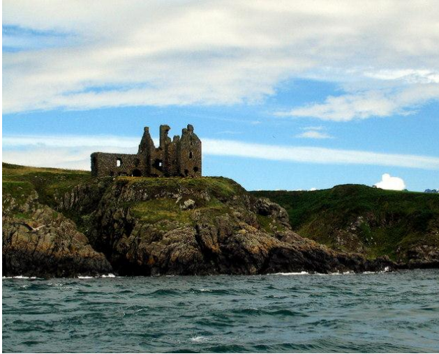
FIGURE 36 DUNSKEY CASTLE, BOUGHT FOR RESTORATION IN 1998 BUT NEVER STARTED 307
