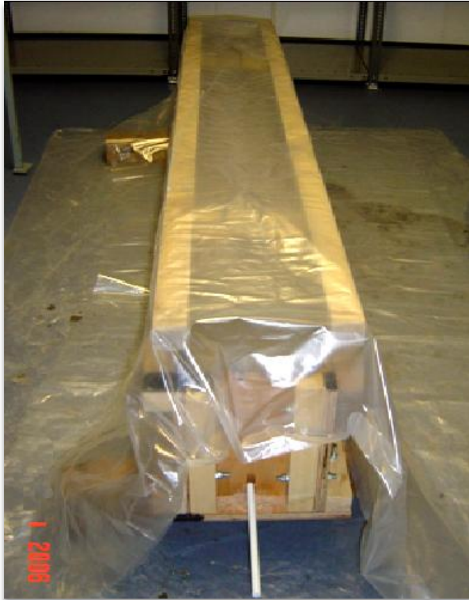
Figure 4.8: Beam covered in plastic sheet after cast
