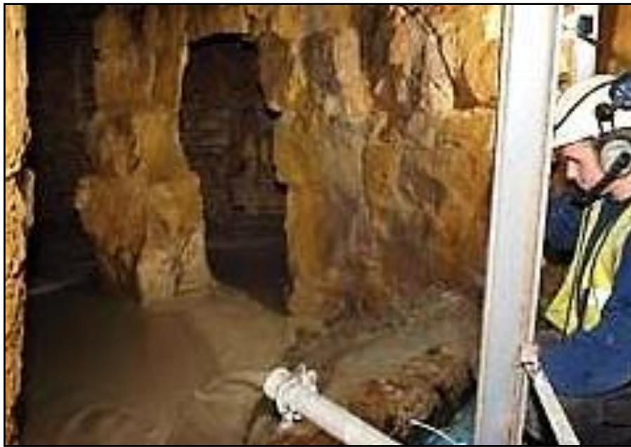
Figure 7.2: Combe Down mine stabilization project ( http://www.foamedconcrete.co.uk/studies_combe.php , January 2010).
