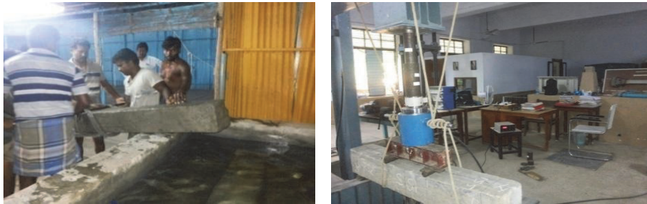
FIGURE 5: Removal of beams from potable water and experimental setup of beam.
