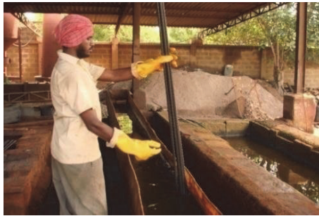
(a) HYSD rebars are cleaned in caustic fluxing
