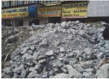
(a) Collection of aggregates from demolished foot-bridge
