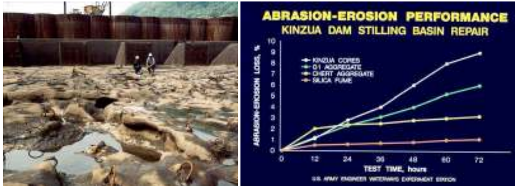
Figure 2 Kinzua Dam: The damage shown is in 1983, after only 9 years. The repair concrete using silica fume (lowest abrasion result in the USAEWES test) is not even being considered for replacement (2012).
