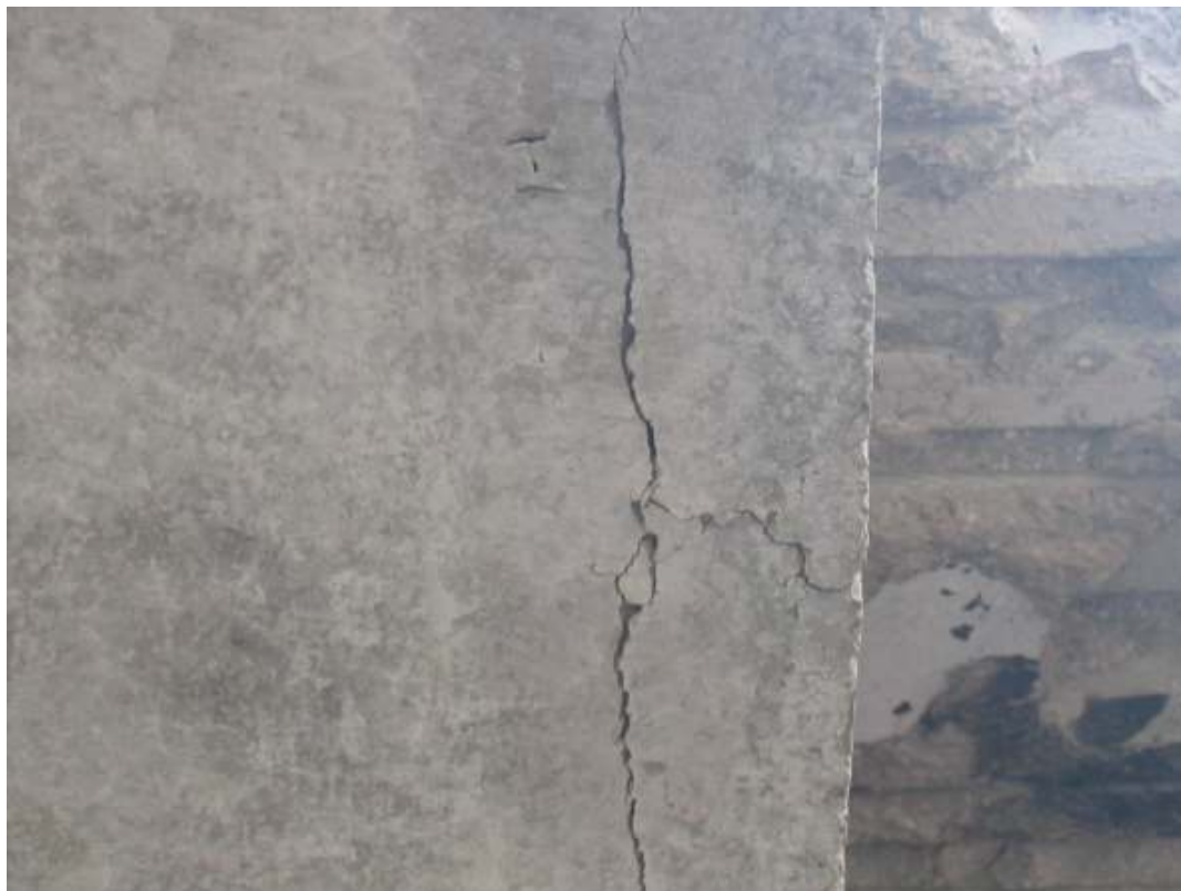
Figure 6 Cracks in a reinforced concrete column
