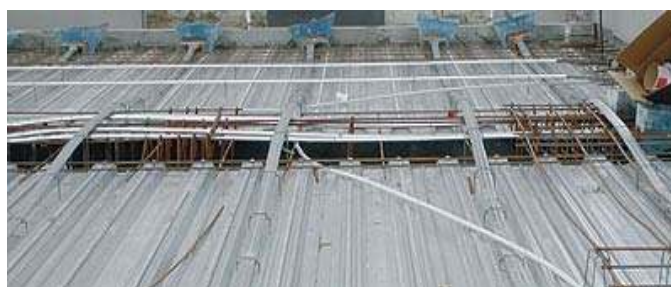
(b) Decking prior to placing concrete
