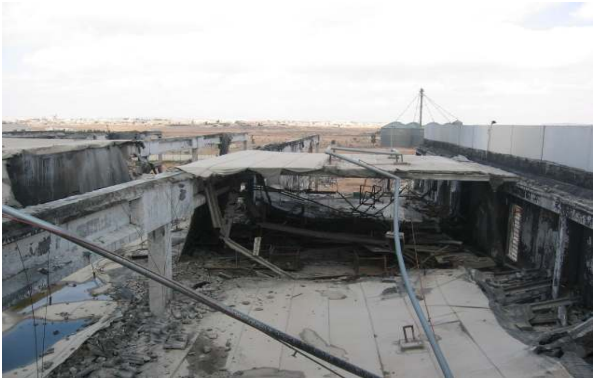
Figure 4 Collapse of slab panels of 1 st floor on ground floor slabs in Zone 2
