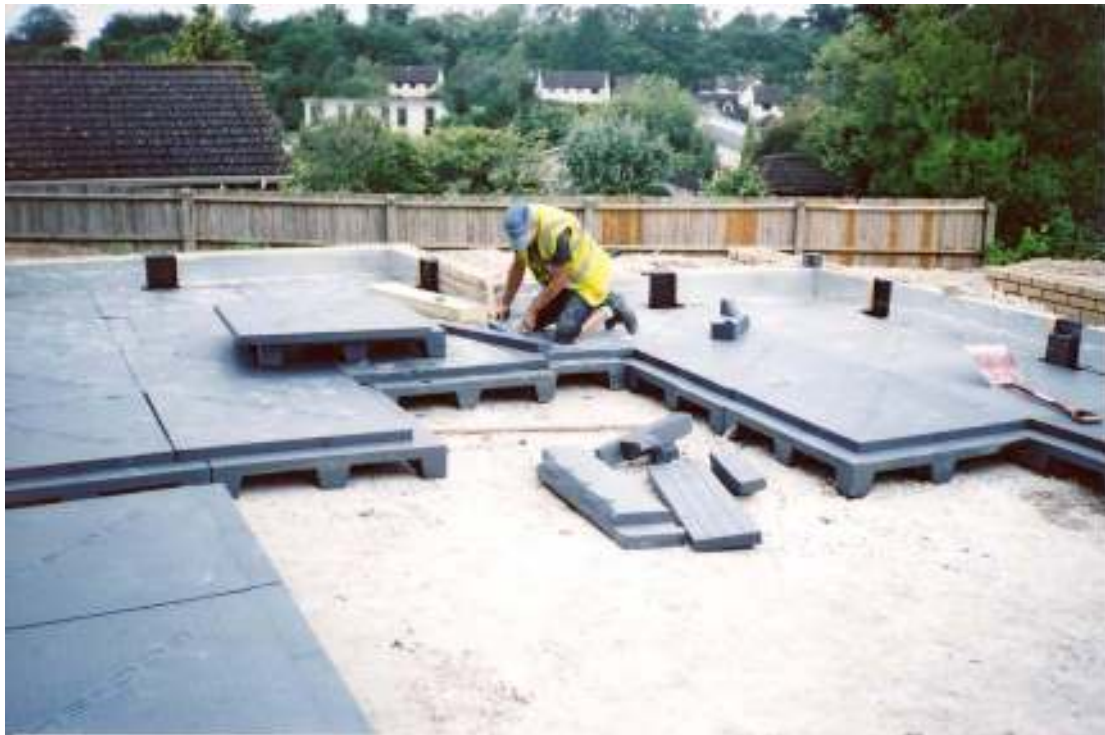
Figure 1 Placing the insulation units
