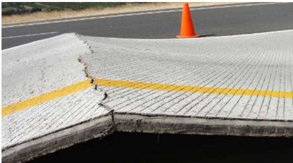
Figure 11 UTCRCP failure
