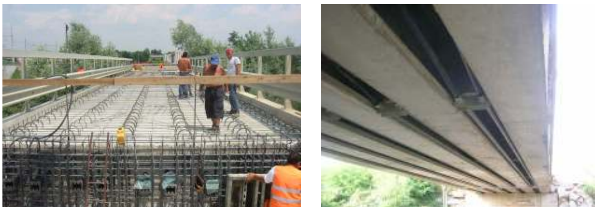
Figure 4 a) Building of new slab connected to the old deck; b) View of externally prestressing
