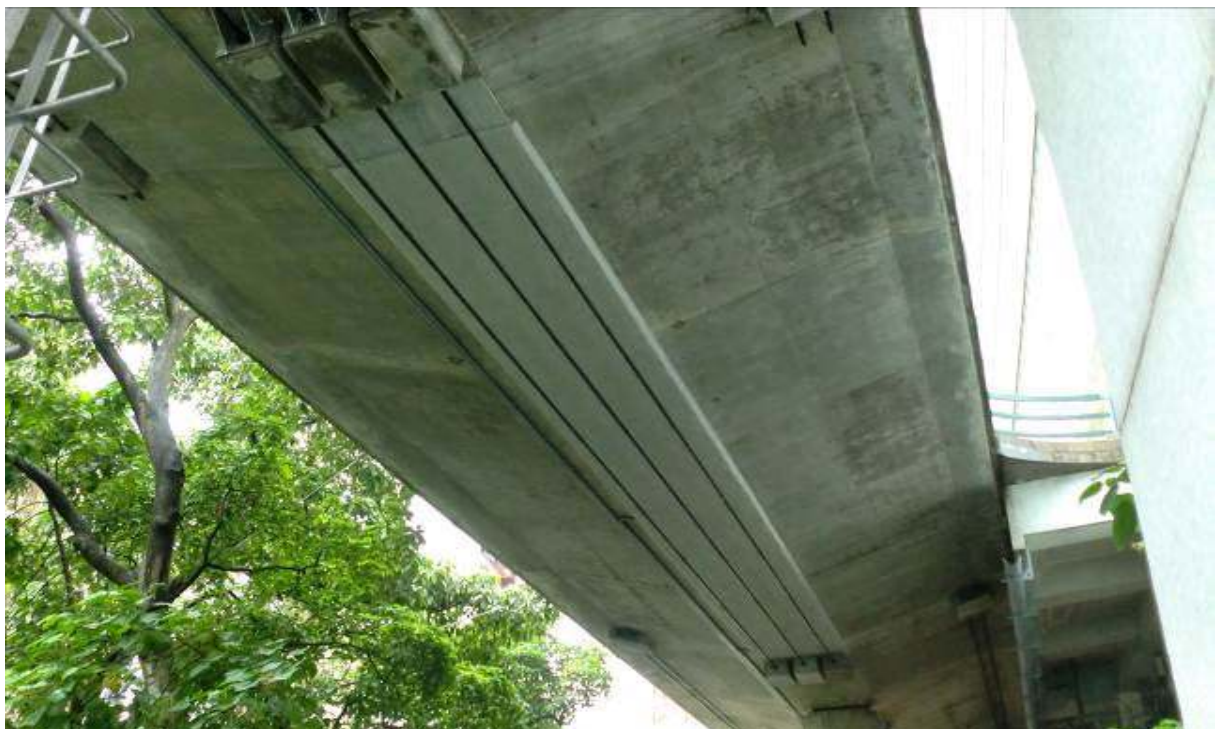
Figure 2 Bridge after strengthening works
