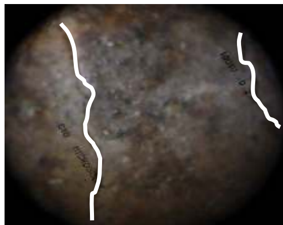
Figure 8 Shrinkage cracking occurrence on plain concrete
