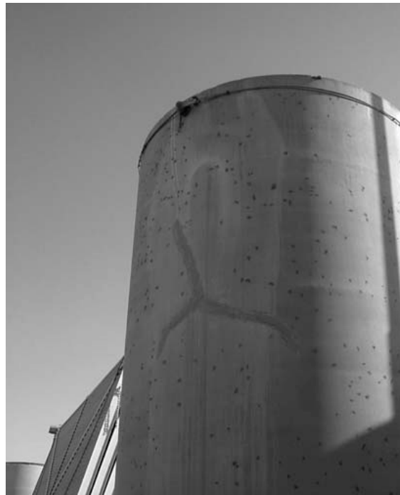
Figure 5 Thermal cracks
