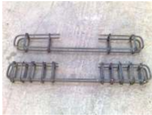
Figure 1 The form of reinforcement used in beams
