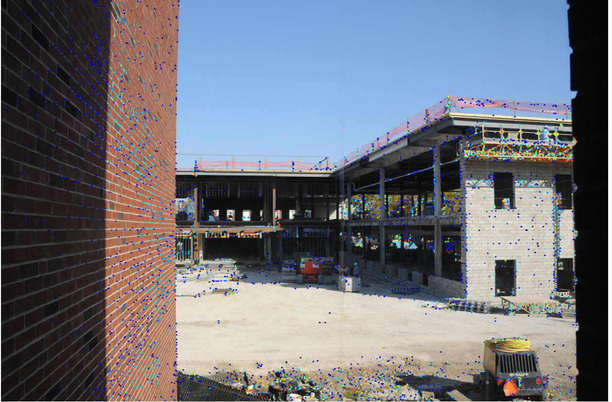
Figure 1: SIFT detector returns 11919 keypoints on a 2144 x 1424 image (SD9 data set). Small dots indicate the center of keypoints while their color shows response level of keypoints
