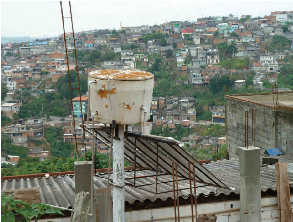
Figure 4.9: low cost DIY SHW in the favela Pretoria, Municipality of Franco da Rocha, Greater São Paulo (Case study 4).
