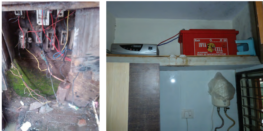
Figures 2.2 and 2.4: Informal electricity connections in Ghatkopar, Mumbai and inverter and battery pack for residential electricity provision, Thane.
