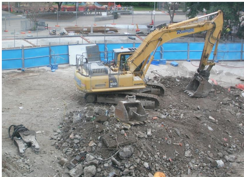
Figure 2: Excavator with attachments
