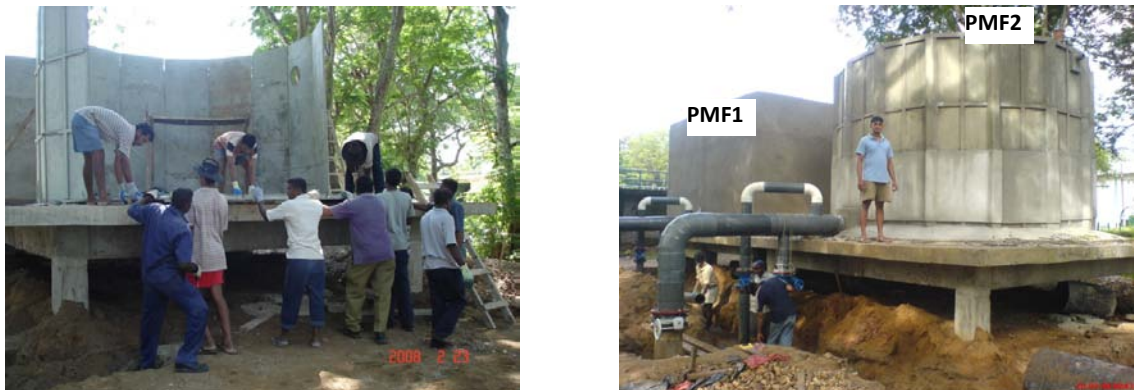
Figure 3: Photos of 4.8 m x 4.8 m RC Tank and 4.5 m Diameter FC Tank
