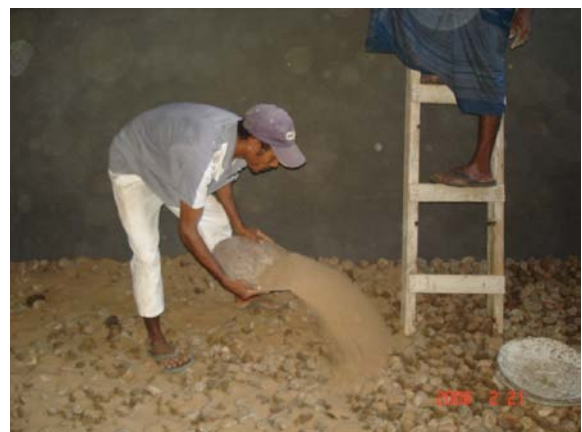
Figure 5: Placing the Pebbles & Sand Mixed Bed Manually
