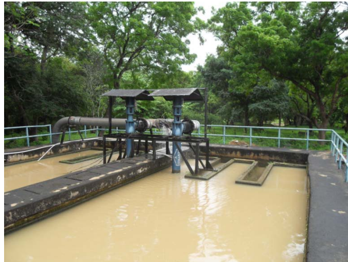
Figure 7: Backwash Water Supply from Sedimentation Tank
