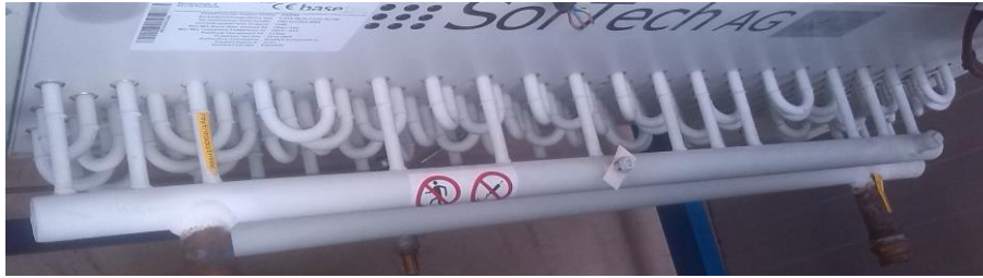
Figure 3.3 Sortech AG RCS 08 - Front water circuits pattern
