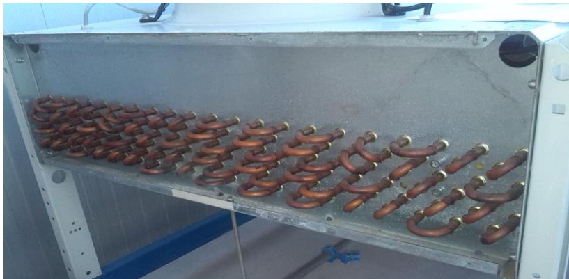
Figure 3.4 Sortech AG RCS 08 - Back water circuits pattern
