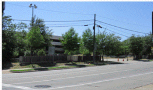
Before condition of Harry Hines at Payne St
