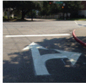
After condition at Wolf St - EB
