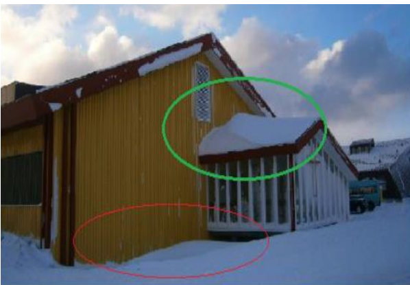
Figure 10: Reference test case to calibrate the snow accumulation simulation on real life observations from Greenland.
