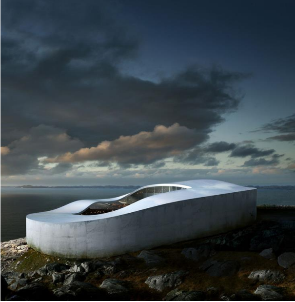
Figure 6: The international operating Danish architecture firm Bjarke Ingels Group (BIG) designed a new gallery in Greenland. The new building for modern Greenlandic art will be located on a steep hillside near the old colonial harbour close to the sea. The building forms a circle around an inner sculpture garden and follows with a nearly constant elevation height the contour of the rugged landscape (picture: BIG architects, available at: < http://big.dk/press/nuuk_146 >).
