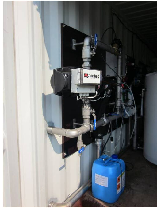
Fig. 7: Amiad pre-filter + biocide dosing
