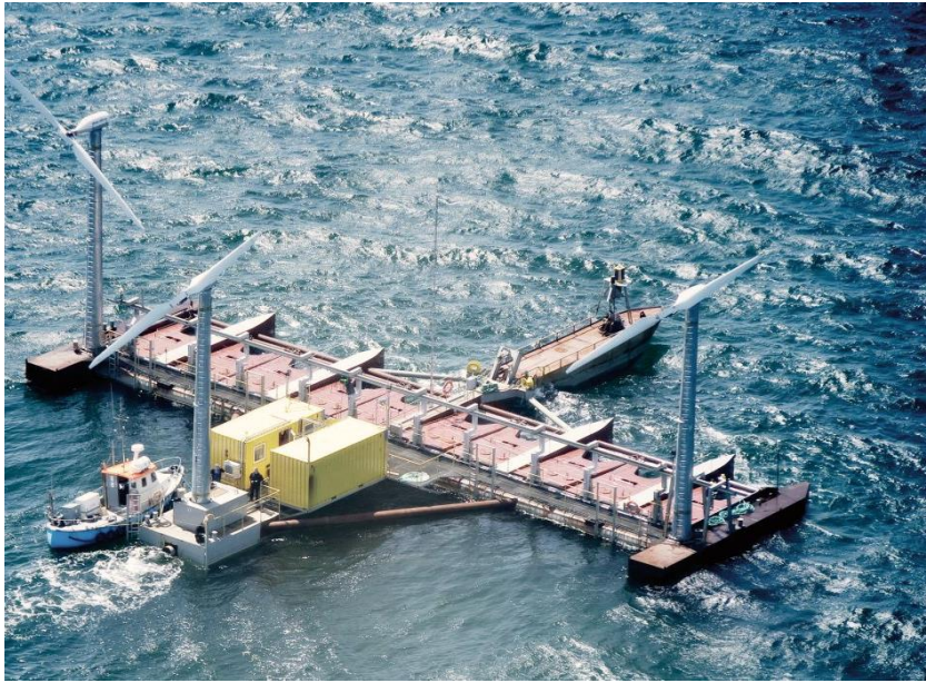
Figure 5. P37 demonstration platform in operation
