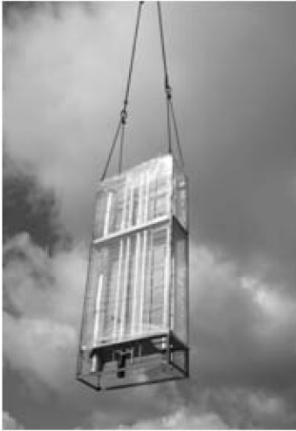
Fig. (1). The prefabricated shaft.
