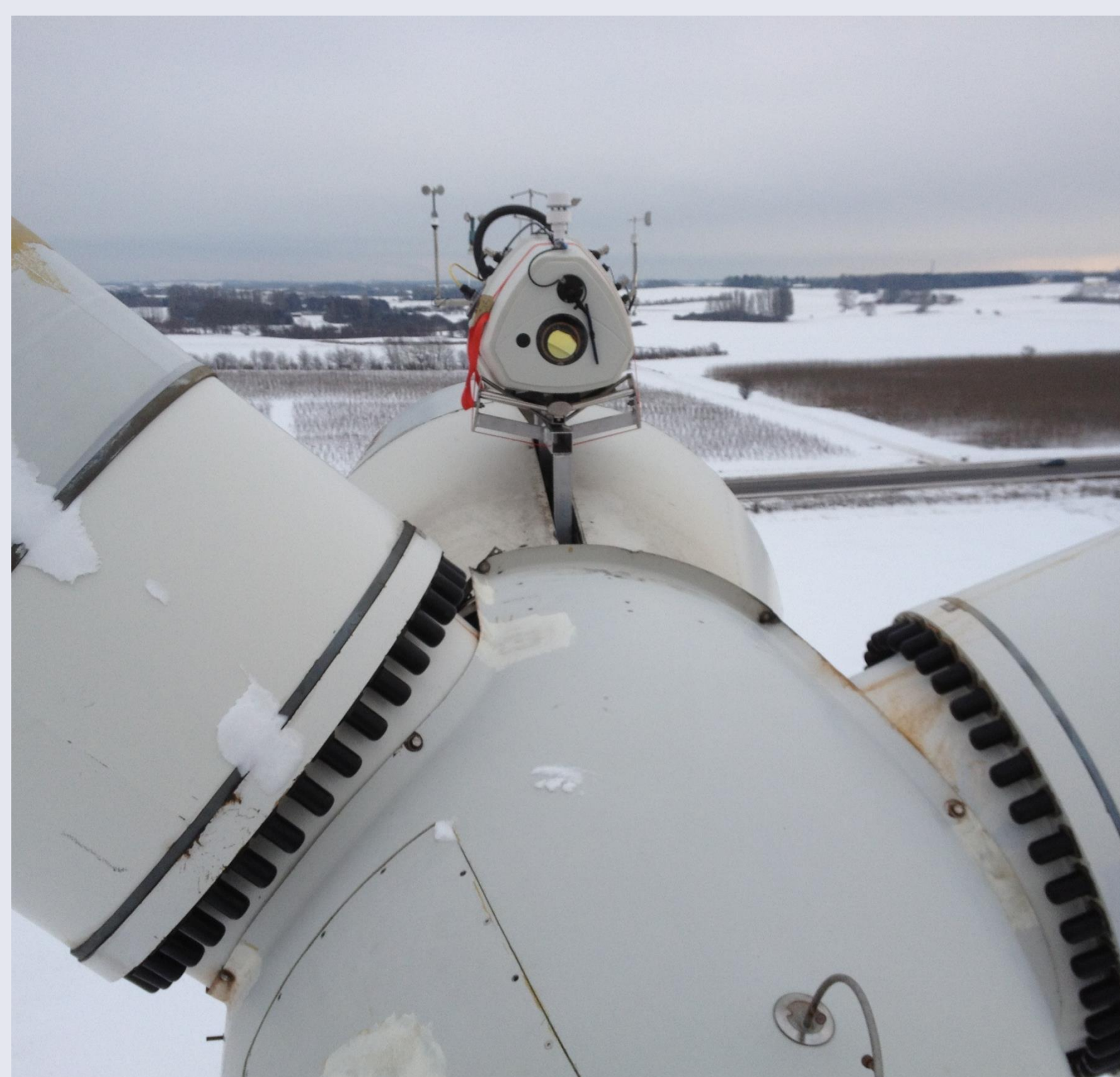
Figure 1: ZephIR DM mounted on nacelle of turbine at DTU Risø Campus
