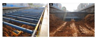
Fig. 5. Working site of the excavation of the Mingdu Station: (a) steel support; and (b) foundation pit
