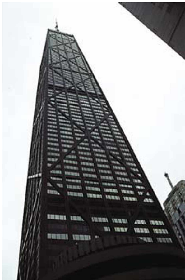
Fig. 1. The use of LSB system in John Hancock, Chicago (Leonard 2007)
