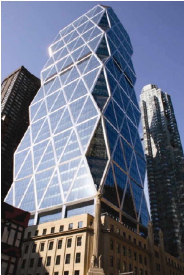
Fig. 4. The use of LSB system in Hearst Tower, New York (Leonard 2007)
