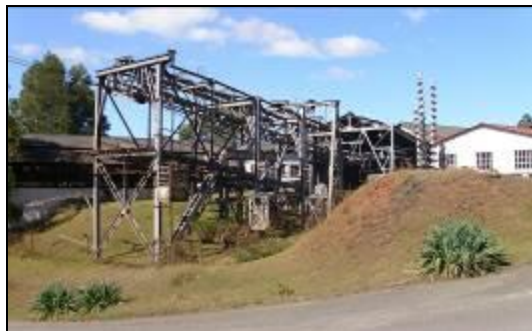
Figure 14. End-station of the cableway in Bulembu for the transport of raw asbestos to Barberton in South Africa. The building in the right is now housing the Bulembu Museum
