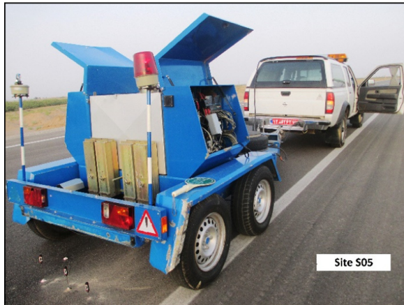
Fig. 3. FWD testing and depth temperature measurements of asphalt layers on a pavement site
