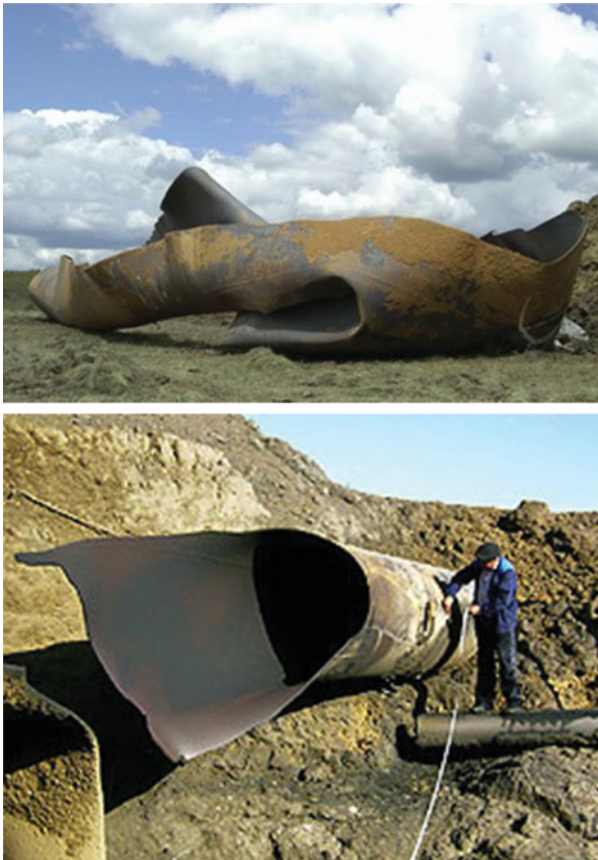
Fig. 2. Breaking-off the Urengoy–Pomary–Uzhgorod pipeline as a result of the gas explosion
