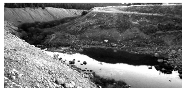
Fig. 14. View of new trapezoidal cross-section in Goksu downstream (November 2011)
