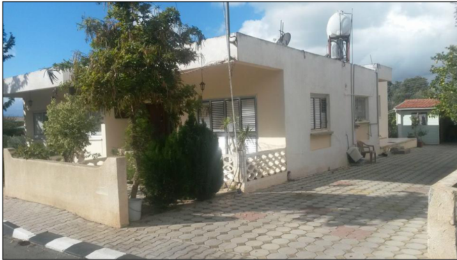
Fig. 9 View of the investigated building
