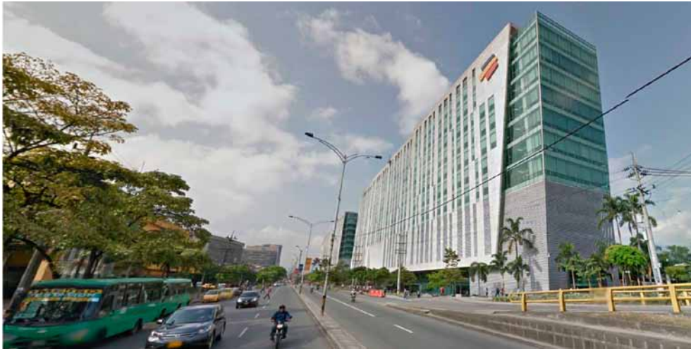
Fig. 16. Bancolombia headquarters in Medellín. This is the largest commercial bank in Colombia. Photo Google Earth, November 2016.
