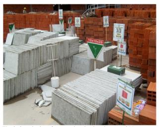
Fig. 8. Organization of construction sites based on visual Management and 5S
