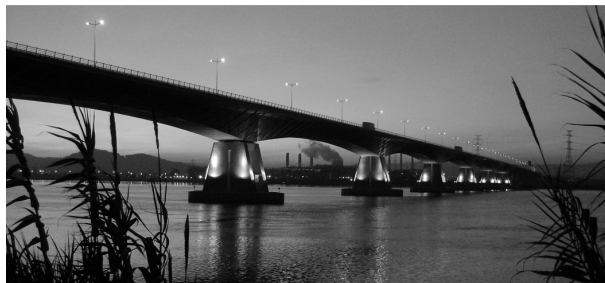
b) Lezíria Bridge (main structure)
