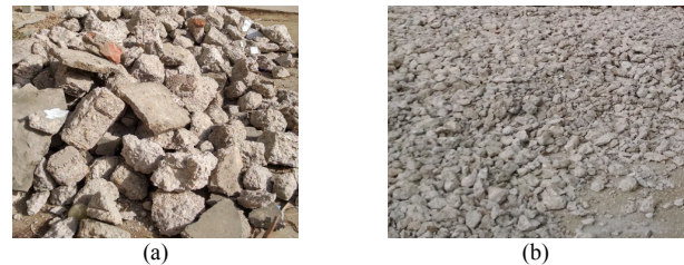
Fig. 1. (a) Old concrete, (b) RCA hammered to 25mm
