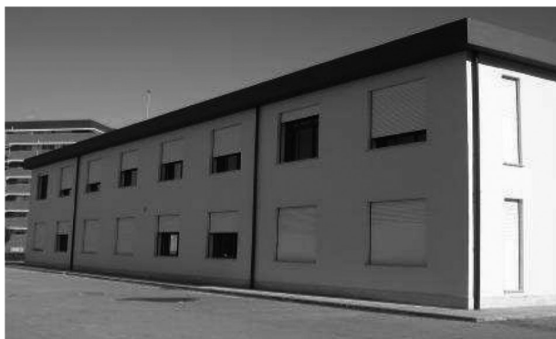
Fig. 6. Example case: school building in Porto (location A)
