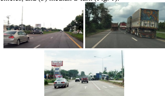
(a) Access-point (b) Heavy vehicle (c) Median u-turn Fig. 1. Factors affecting four-lane highways' capacity in Thailand
