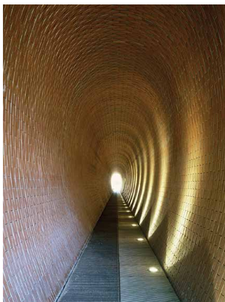
Fig. 1. Josef Pleskot, AP Atelier: Tunnel in the Deer Moat, Prague Castle, 1996–2002. J. Malý photo
