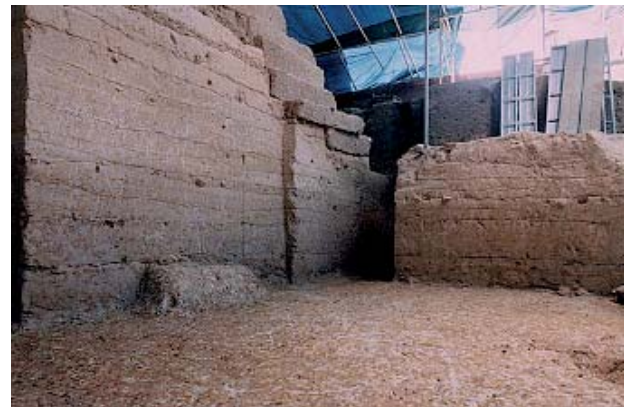
Photo 5. Trenched EW section (note the horizontal layers)
