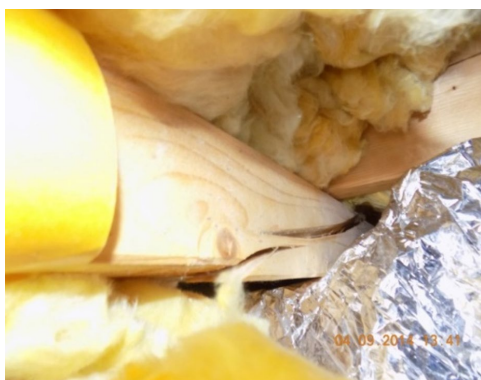
Fig. 14. Splitting of the bottom grains in the roof rafter at the bracing element, double rafter elements (two panels) cause distribution of loading to sound neighboring element and elimination of excessive deformations, failure damage of joist in the floor over the second floor.
