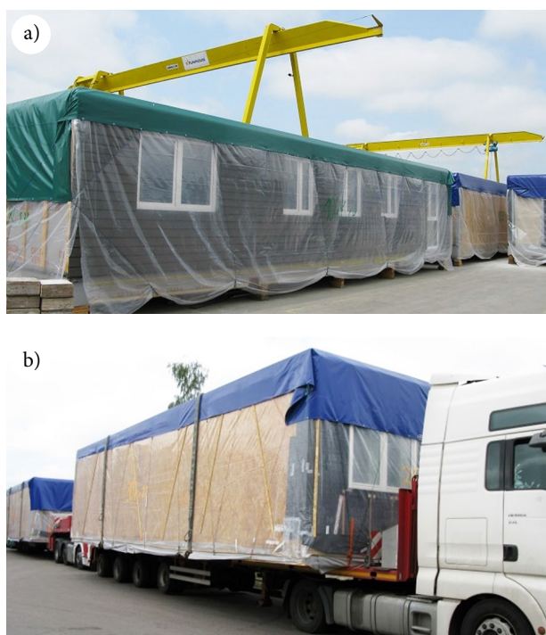
Fig. 9. Loading and transportation to the site
