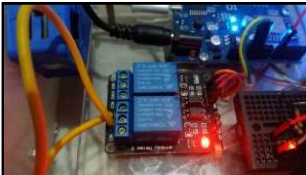
Figure 10.Testing of 2 Channel Relays
