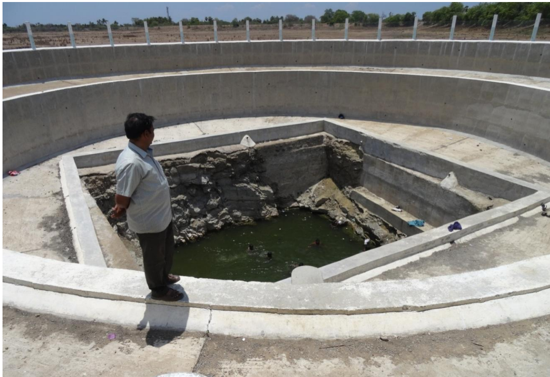
Figure 6. Recharge Shaft, Ulagapuram, April 2017, fence opened and people bathing.
