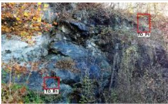
Fig. 3 Overview of Torrente Orba site
